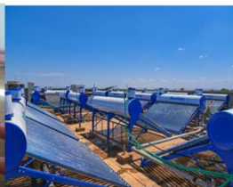
RENOVATED SOLAR WATER HEATING SYSTEM
