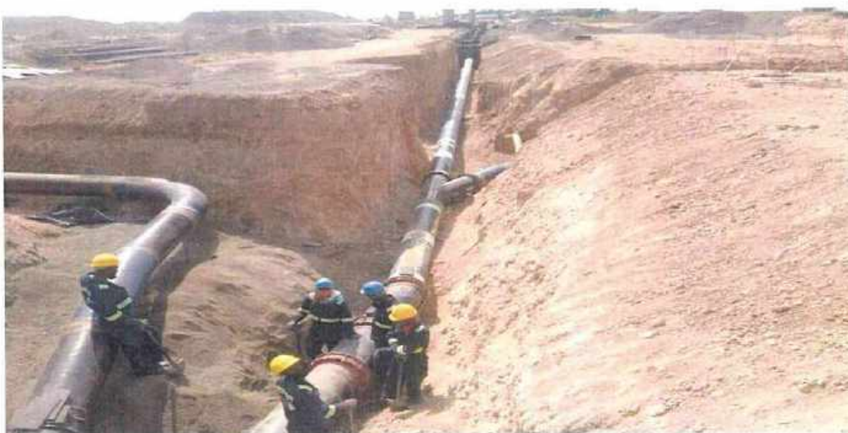
Pipe laying for Solid Waste network along Green Transit Corridor
