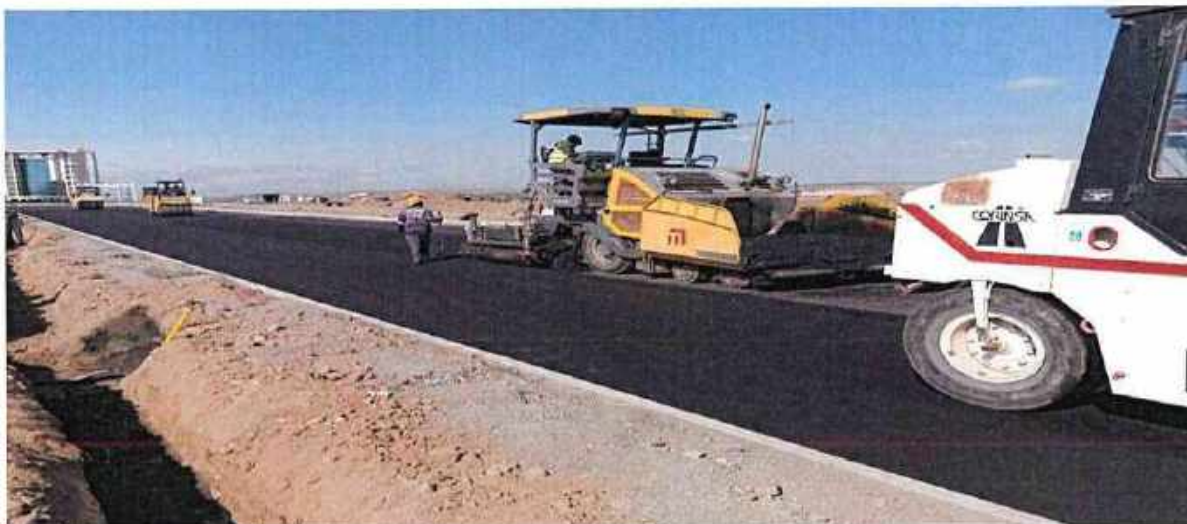
Asphalt laying at LR01
