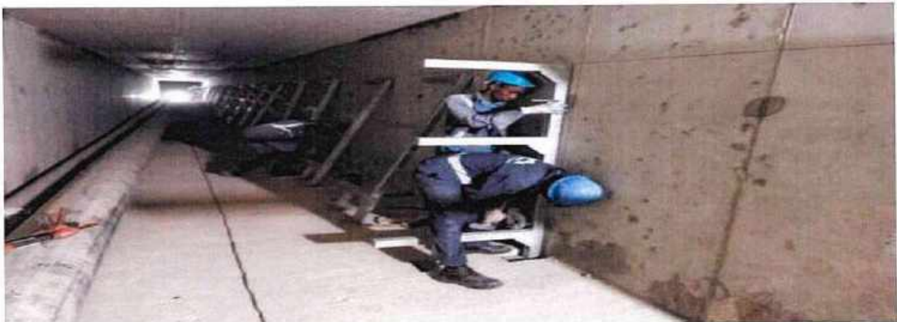
Installation of Utilities Racks inside Tunnel C situated along Auto boulevard.
