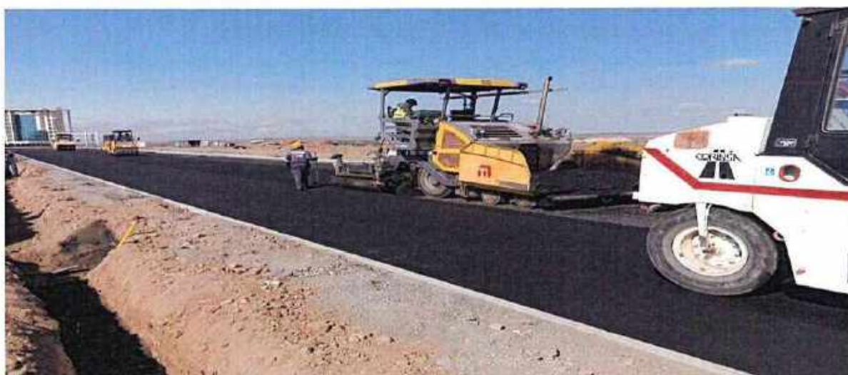
Asphalt laying at LR01
