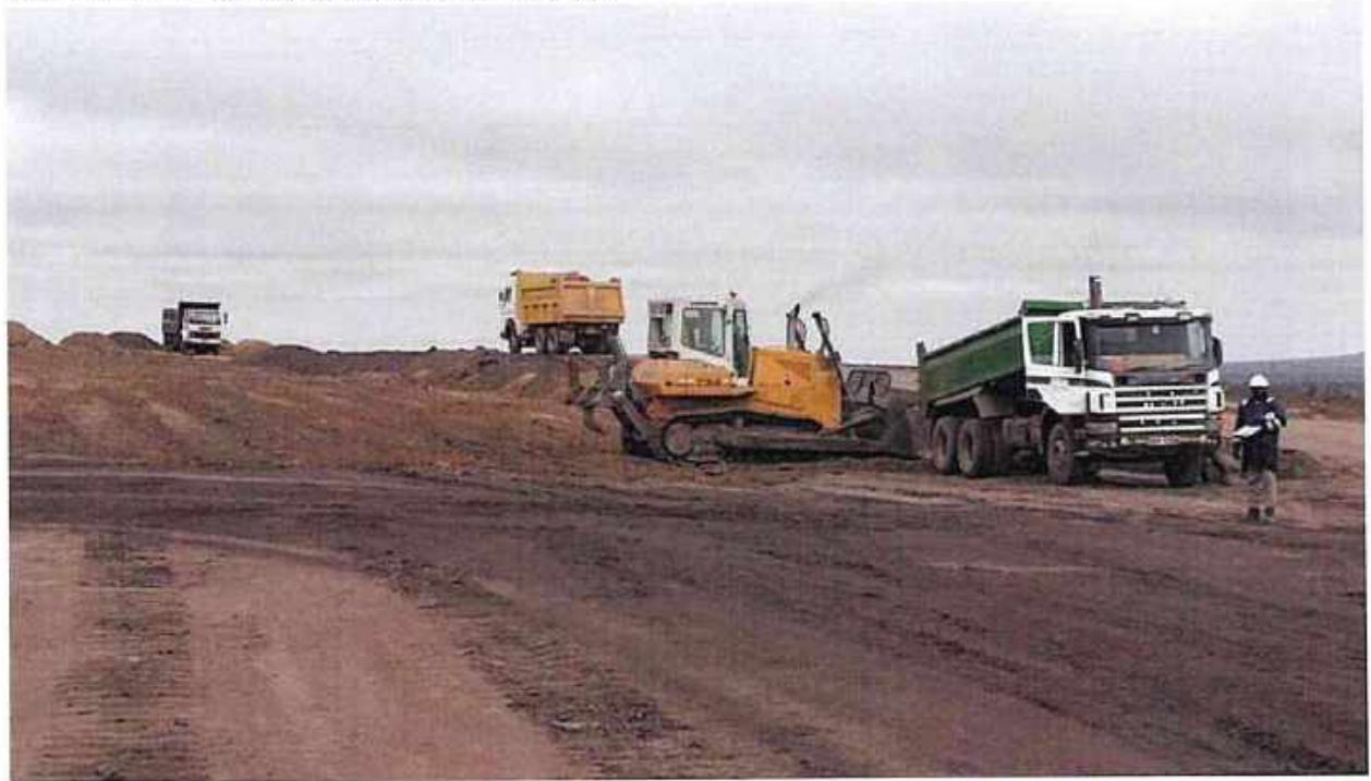
North berm-dumping of material and shaping
