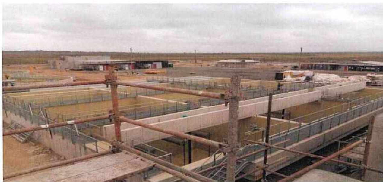
MBBR tank under construction
