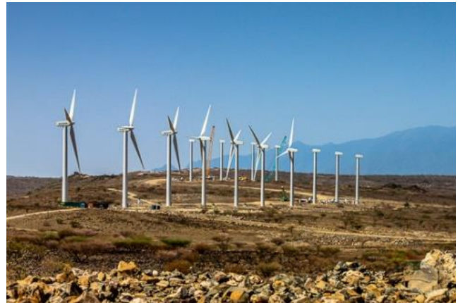
Turkana wind mill project
