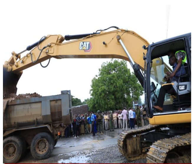
Building of road linking Kenya and Tanzania
