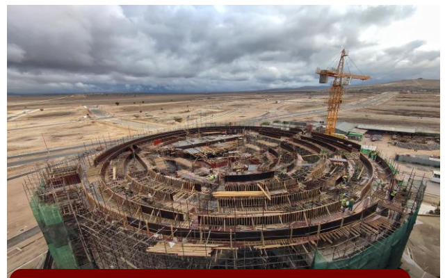
Ongoing construction of Konza Conference Centre
