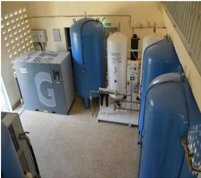
To meet the rising demand for CCU, Mwai Kibaki Hospital constructed and operationalized an Oxygen plant with a capacity to produce 1,500 litres of oxygen per minute, 2,160,000 in 24 hours, and has 18 ports filling station with an ability to fill in 72 oxygen cylinders in 24 hours. The Hospital also acquired a 3000-litres bulk liquid oxygen tank in the FY 2021/22. The facility is supporting the provision of oxygen to other health facilities within the region.
